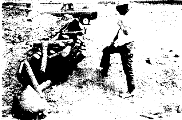
Fig. 9.6. Collapsed entrance facing away from ground zero, at 15 psi. The blast winds had scoured away most of the covering earth, and the earth had "flowed" away from the center of the shelter, pushing the upper part of the entry in a direction perpendicular to the radius from ground zero.
